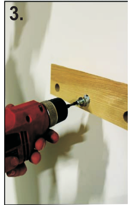
3. Secure the screws tight into the hole drilled in the wall with the help of drill
