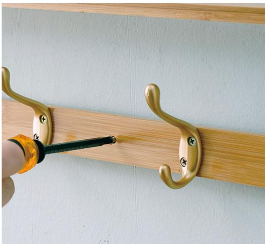
20.If you are afraid that it is not firm enough, you can also install it with expansion screws in the middle hole of the hook stop strip
