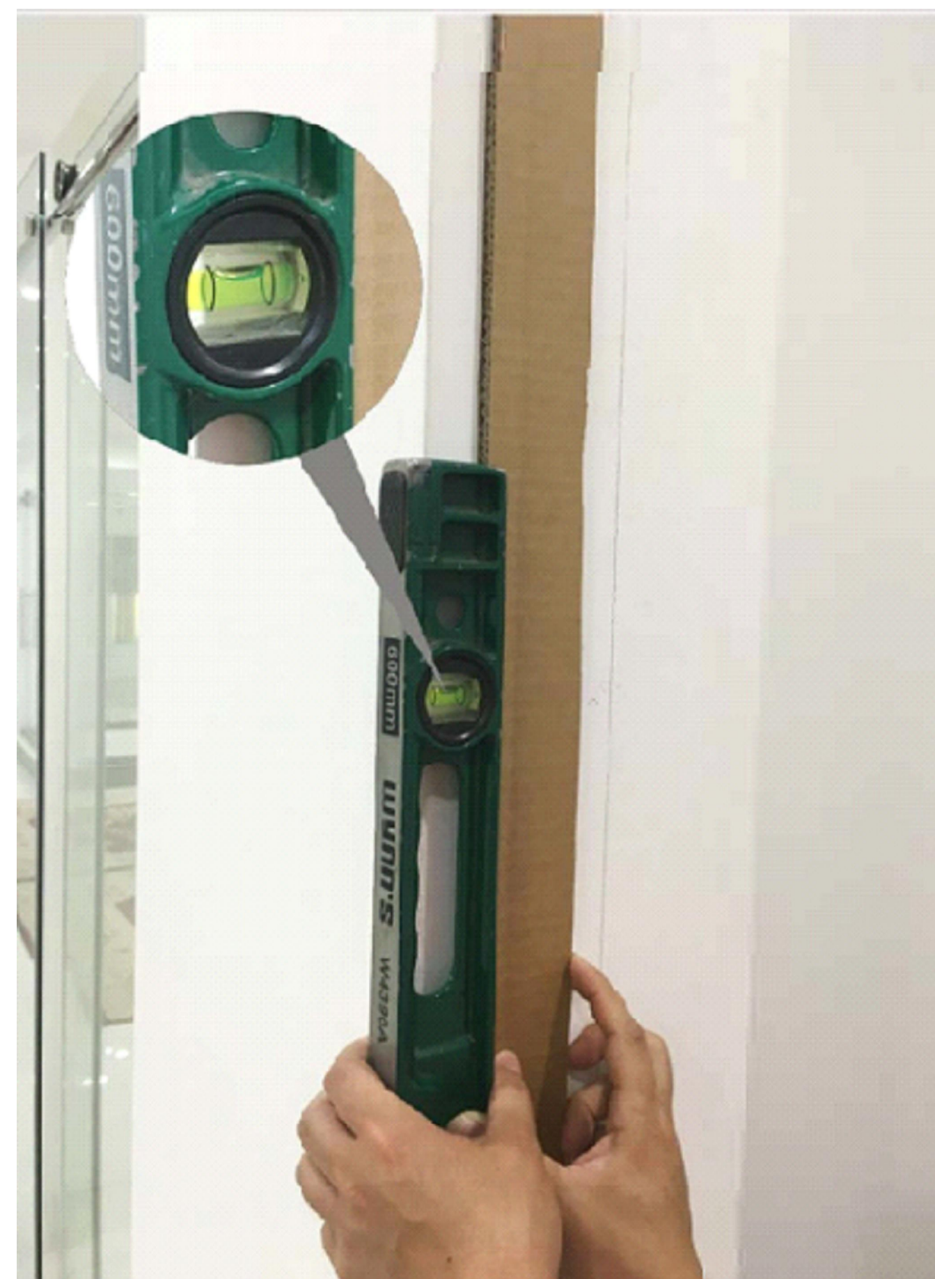
2. Make sure to level the template.
