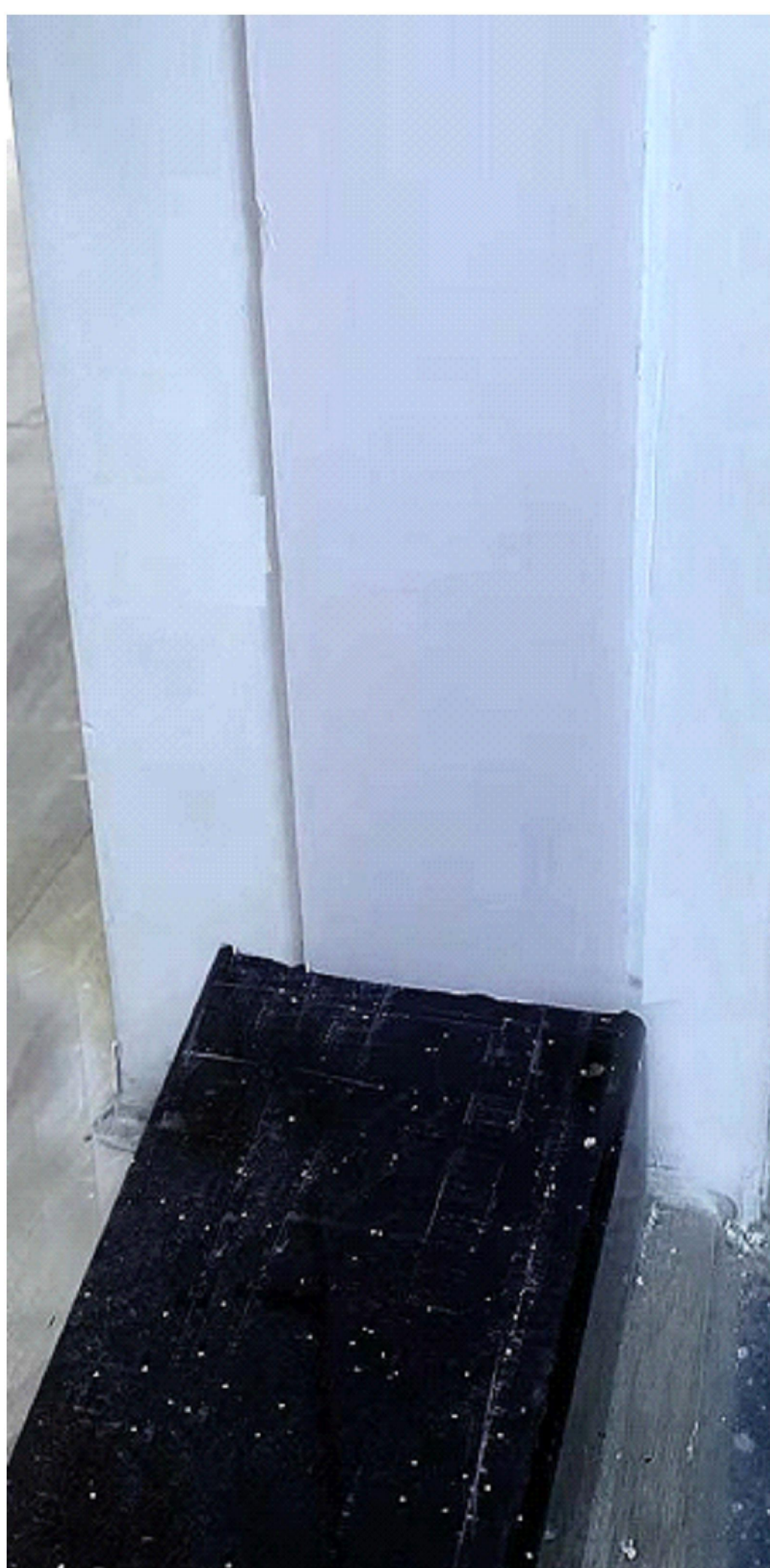
1. Lean the template on the wall.
