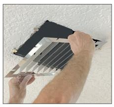
**8.** Install inner baffle under magnets installed.
