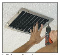
9. Tighten self tapping screws with magnets flat to the ceiling. Tighten enough to bring vent box tight to the ceiling, DO NOT over tighten and strip the screw. Position baffles as needed. They work the best as open as possible.
