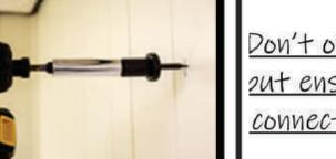
Starting at the center hole using your drill or ratchet you will drill the center layout hole, then set your spacer and bolt,
