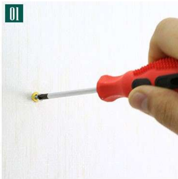
Install the expansion screw into the wall
