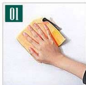
Wipe the wall clean with a dry cloth
