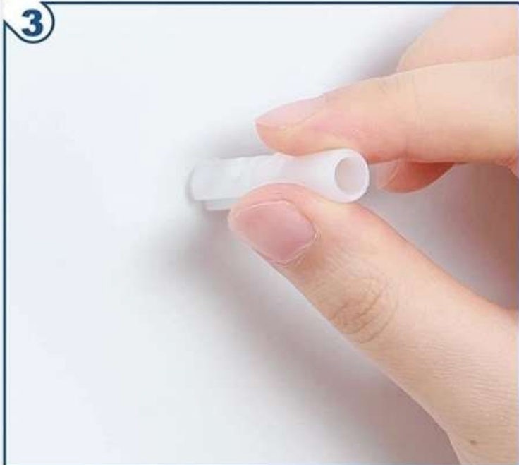
3 Insert expansion bolts into holes
