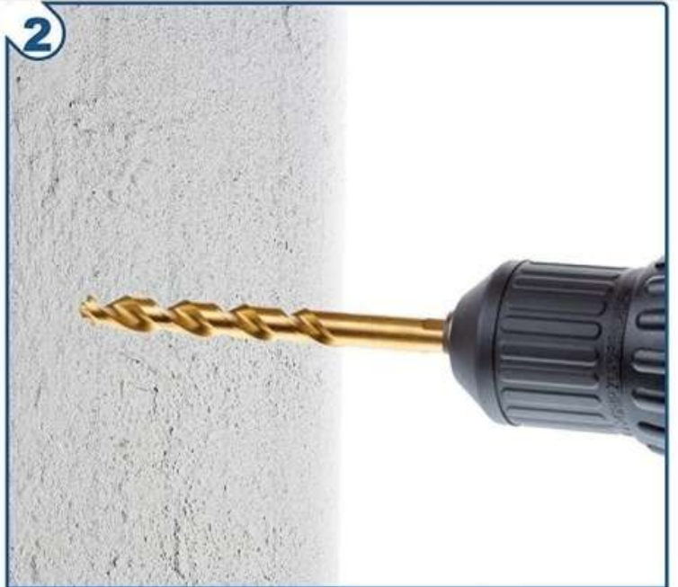
2 Punch holes with M8 drill.
