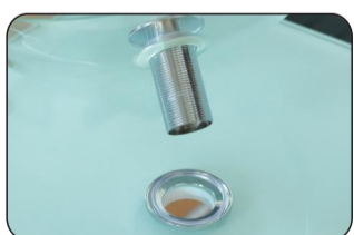
Align the sink with the drain hole and set it up (Thread seal tape five or six laps)
