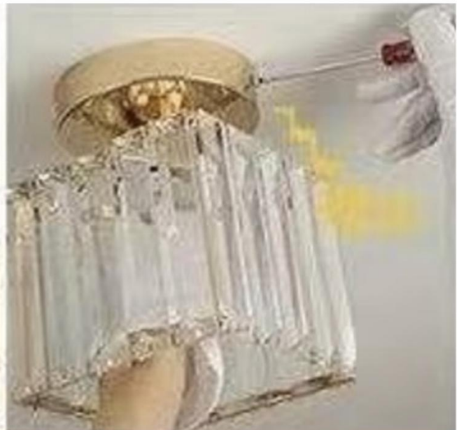
4. Fix the ceiling plate of the lamp to the hanging board with screws
