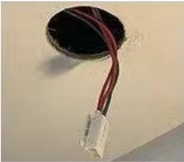
1. Open holes for wiring
