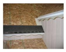
Place piece of flashing #3 as shown and place starter strip over it.
