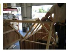
For the **10x18 Mansion** you will add 4 angled pieces to hold the roof as shown in pictures number 85 & 86. In the 8x16 this roof sheeting is held by a V-channel roof brace.
