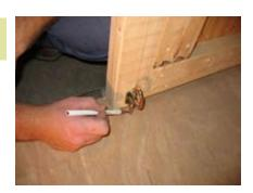
Fasten 2x4 for door and fasten barrel bolts on top and bottom. Draw a circle where the bolt will slide into. Drill a hole for it to go into.
