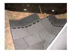
Snap a chalk line down the center of each valley. Place shingles in this area to fit.
