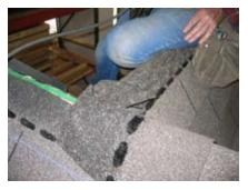
Continue installing and cutting ridge cap to fit.
