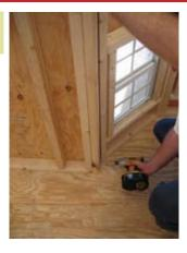
Install the 2x3 on the end of panel O as shown in this and the next picture.
