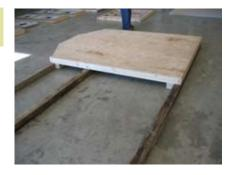
Lay bay window side of the floor section on top of these 4x4's. Note how the 4x4s are positioned against shipping blocks. Center 4x4 is to be aligned with the marked area.
