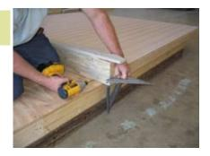
Set up panel A. Be sure to keep the bottom of the siding pushed in.
