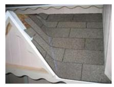
Run shingles to the top. Snap chalk line down the center of the valley. Install shingles on dormer (cut to fit).
