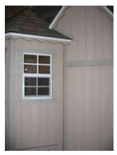
Install trim on the backside of teh turret, Also note the small trim piece that is covering teh flashing by the shingles. (you had to remove it to install the flashing).
