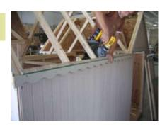
Fasten small OSB strip along the bottom backside of the turret side.
