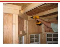
Remove braces since walls are now stabilized with the trusses and sheeting.
