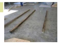
Lay (2) 4x4x16 and (1) 4x4x14 pressure treated runners as shown...the floor will line them up in the correct place.
