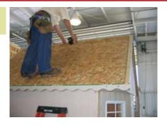
Install the first piece of sheeting on the bayside. Refer to sheeting exhibit for sizes. make sure the truss measurements on the top match what was premarked on the bottom.
