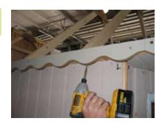
Fasten trusses underneath through the 2x6 as shown.
