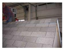
Run shingles up the small side over teh valley. Then chalk the center and cut long side shingles to match.
