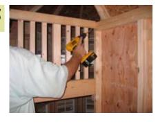
Fasten the 2x6 in between the trusses, keep to the top toward gusset.
