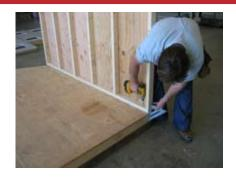
Install panle B as shown. Fasten in the front then the back.
