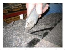
Cut shingle to fit over. Note using the hook knife.
