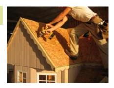
Hold V-channel into place. The 10x18 will have 4 additional braces for the roof (it is a larger roof).
