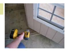
Do this same thing for panels K thru N. Be sure to follow teh diagram and install in the correct pattern. Otherwise the gingerbread will not match as well.
