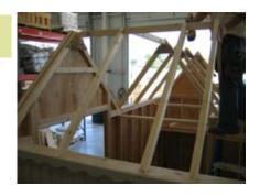
Install rear truss onto T-bar, in premarked spots.
