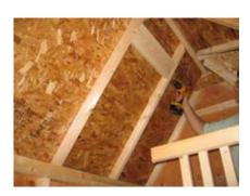
Fasten the loft railing post onto the 2x6 and the railing.
