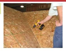
Now fasten the loft underneath all the way around.
