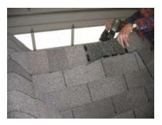
Start adding ridgecap from turret back to teh roof line.
