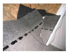
Install shingles over these. Leave small place between shingles so that water is not trapped.
