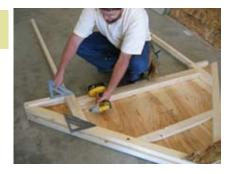
Fasten 2x3's as shown to panel T. Be sure to keep even and all the way to the top.
