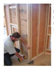
Fasten the bottom of the siding to the floor.
