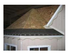
Next place starter strip of shingles. (refer to shingle package on how to cut). You basically cut off teh tabs and use the back side of a shingle.
