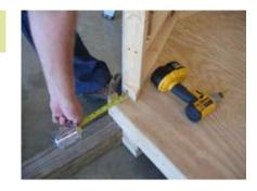
Install panel. Fasten panel D to panel E where it is marked.
