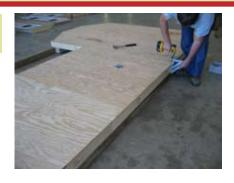
Make sure it is even on the ends before fastening. Then add plywood to the center after fastening turret section.
