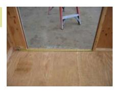
Make sure there is 34" in between the 2x3s for the door opening. Otherwise the door will fit too tightly. You may have to loosen the walls and move slightly to get this measurement at the bottom.
