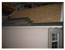
Place starter strip and fasten shingles on bay window side. Install all the way to the top.
