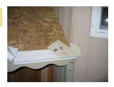
Place and fasten flashing #5 on porch roof by turret side.
