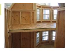
Install braces as shown to stabilize walls til trusses and sheeting is installed.
