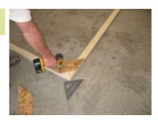
Assemble trusses for the bayside window part of the house. Be sure to keep the top even. Use black screws for this. Be sure to fasten the correct tops together.
