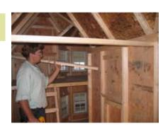
Install loft railing. Be sure to add plenty of screws to hold in place.
