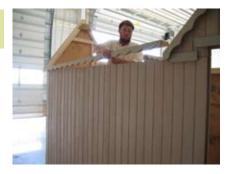
Fasten the 2x6 with gingerbread to the top of panels Q & R.
