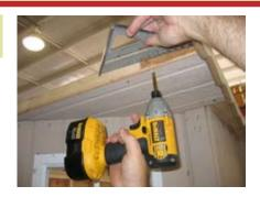
Fasten into the bay windows. This will tremendously strengthen the bay window.
