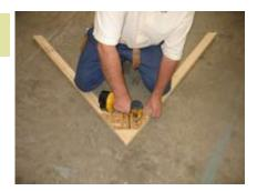
Fasten truss in premarked spots. This shows the truss being fastened to the side of panel I.
