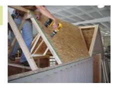
Install this sheet of OSB. Make sure the truss measurements at the top match those at the bottom.
