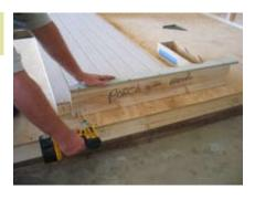
Fasten bottom of the siding to the floor. Be sure to do this all around.
