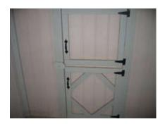
Fasten 3 door latches (one goes on the inside of the top door). Install turner knob to close the door.
