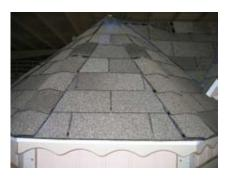
Cut ridgecap 6" for the turret. The smaller size will give it teh correct dimensions. Take these all the way to teh top. (further than shown)
