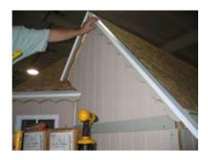
Install dripedge all around the edge of the building. Note the hand is resting on the dripedge.
