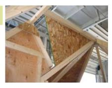
This shows an inside out view of the piece. There will be a piece (2x3) added to hold this sheet in place.
