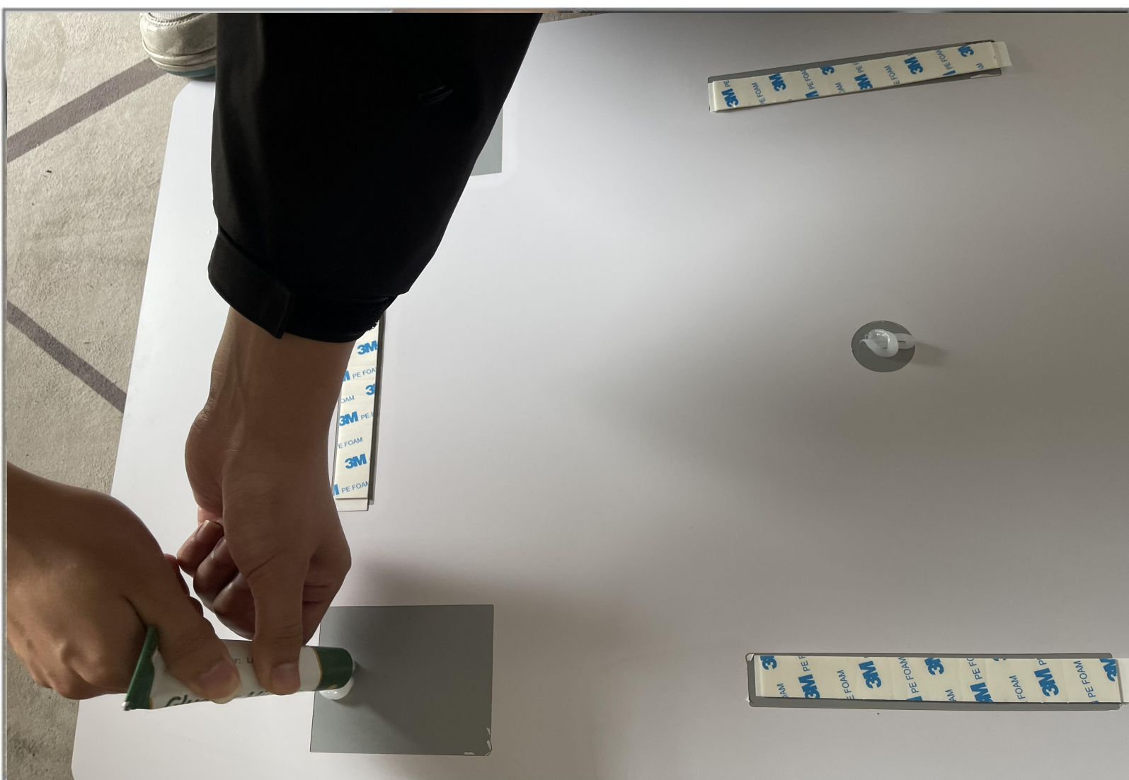
3.Squeeze appropriate amount of glass glue on the round anchor point, glass tape full of dots higher than double-sided tape.
