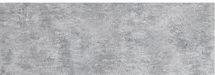
Concrete wall surface
