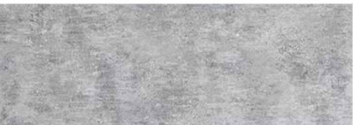
Concrete wall surface
