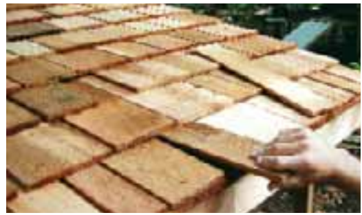
116. Next, time to install Filler Shingles to completely secure gazebo roofs and hide roof seams. Starting on bottom row of shingles, push a Long Filler Shingle (5 1/2" wide) underneath shingles directly above it until end is flush with bottom shingles.
