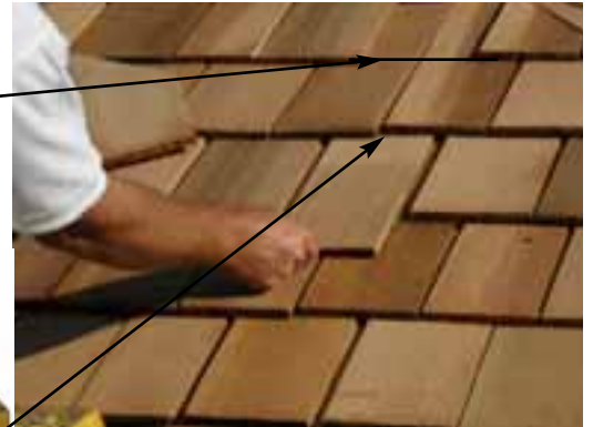
116. Next, time to install Filler Shingles to completely secure gazebo roofs and hide roof seams. Starting on bottom row of shingles, push a Long Filler Shingle (5 1/2" wide) underneath shingles directly above it until end is flush with bottom shingles.
