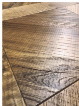
SPLITS IN TIMBER/ SAW MARKINGS
