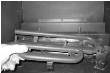
Burner Removed
