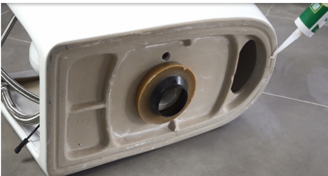
10. Apply a layer of silicone sealant to the base of the toilet. (The glass adhesive in the picture needs to be purchased by oneself.)
