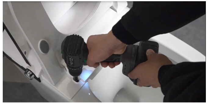
7. Unscrew the screws on the toilet seat
