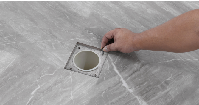
4. Put the screws into the holes.
