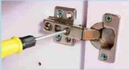
The door seam is too large
