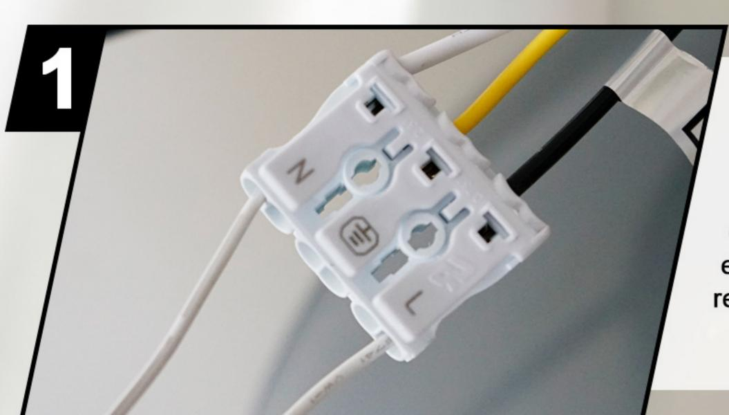
Before connecting the new remote control, it is necessary to disconnect the zero and live wires before reconnecting them. This is to clear the data left by the previous remote control and enable the fan to obtain data from the new remote control.
