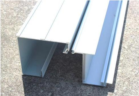
**FIRST:** Lay the hanging channel and front fascia parallel and evenly on a flat level non-abrasive surface or slab. Make sure both front fascia and hanging channel rails remain even and flush together by taping every 15" across span.
