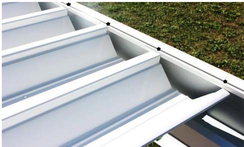
**THIRD:** 12" marks will be needed during future STEPS for locking-in roof panels in the correct location to ensure water-tight connection.
