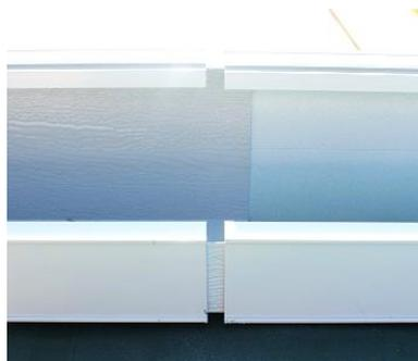
**STEP 4:** Secure splice using 3/8” socket drive and twelve 1/4” x 3/4” Tek screws at 1”, 11”, 13”, and 23” from ends of splice. Caulk all connections and ends generously.
