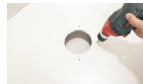
Mark the 4 positions for drilling, then drill holes at the marked spots
