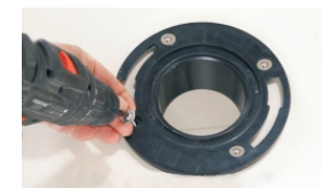
Align the PVC flange ring with the 4 small holes, and tighten the 4 screws to fix it
