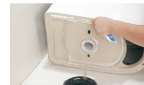
Apply installation adhesive along the bottom edge of the toilet. (Apply the glass glue and let it dry in two hours)
