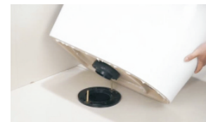
Align it with the sewage outlet, place it down and apply anti-mold glue around it
