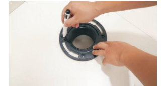
Slip the pvc flange ring over the floor drain outlet
