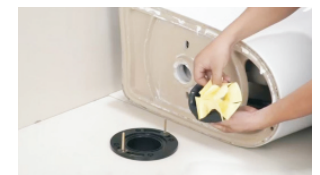
Press the flange ring tightly against the toilet drain outlet
