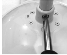
reinstall and tighten stopper screw
