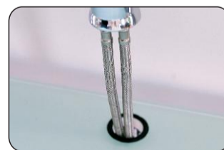
Pass two waterlines through faucet hole of countertop & adjust faucet
