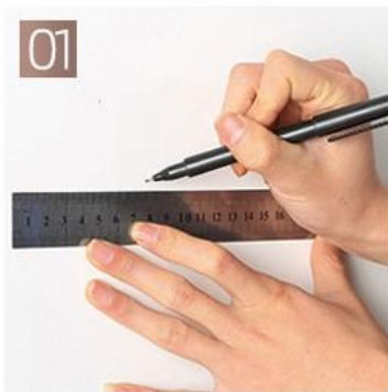
Align the punching position on the wall
