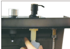
02.Installation of fixed soap dispenser
