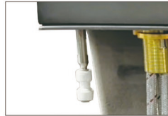
03. Tighten the screws and pipe connector
