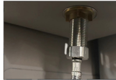
03. Connect the cup washer with the hose
