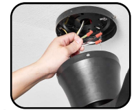
12 Connect ground wires, live wires (BLACK) and null wires (WHITE).
