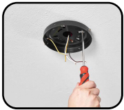
10 Tighten the base.
