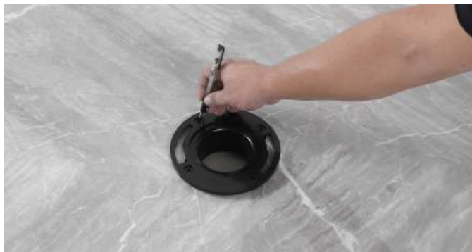
2. Place the fixed disk into the drain outlet and mark the screw hole positions.
