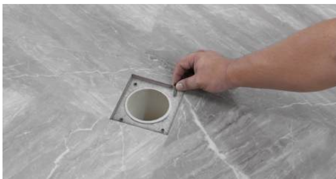
4. Put the screws into the holes.
