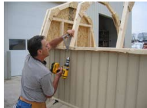
Use angle square as shown to make sure the truss is flush on the outside of the 2x6 and secure with 2 1/2" screws.
