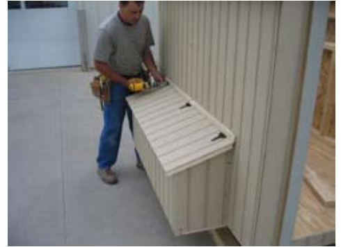
Now install the lid with the 3" t-hinges as shown.
