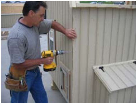
Secure all corners with 1 1/4" screws, every 6" to 8" .
