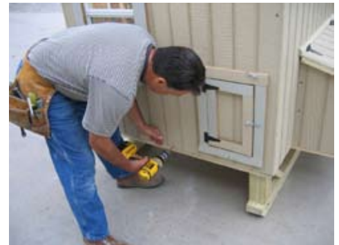
Secure outside bottom edges, with 1 1/4" screws every 6" to 8" .
