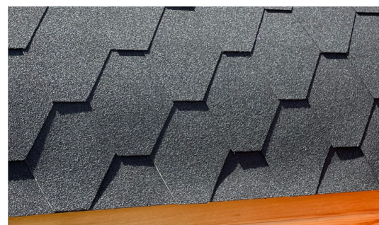
Shingle strip honeycomb pattern on a barrel sauna
