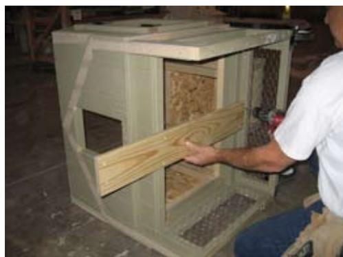
Install the chicken ramp. Secure with 2 1/2" screws. Two in the back and two in the front.
