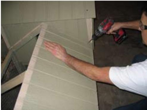
Next install the roof on the lower section. Secure with 1 1/4" screws.
