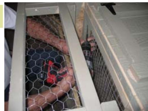
Secure floor with 2 1/2" screws as shown.
