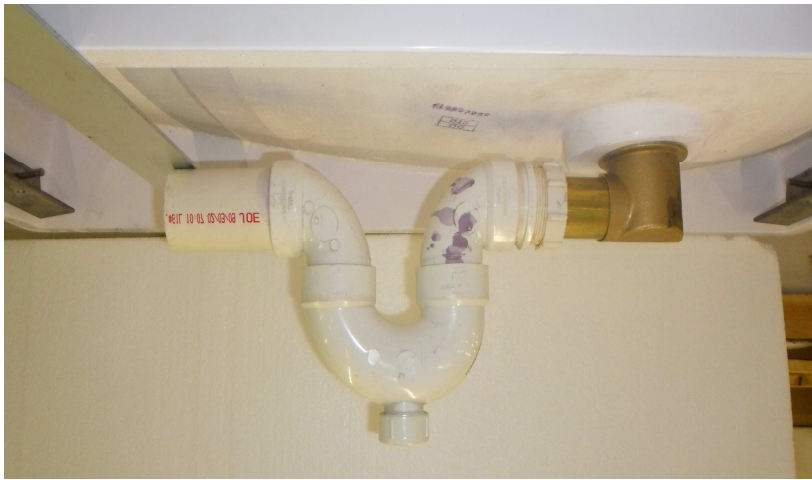
Tub shoe and P-trap connections. Suggested pipe is 1-1/2" diam
