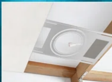
3. Seal the ceiling with gypsum board
