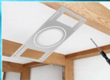
1. Securely fasten the mounting plate with screws
