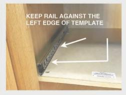
Holding the template in place with both rails up against the left and right edges of the template, as you did on the right side/rail, drive a pan head screw into the center of the *oval* holes in both the front and rear L-brackets of the left rail. Remove the template.
