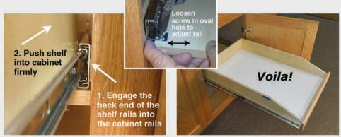
• The end of the shelf rails are placed into the plastic guide clip of their corresponding cabinet rail. If the shelf seems to tight or loose, loosen the screws in the oval holes of the left rail L-brackets and nudge the rail to the right or left as needed and re-tighten. Re-test the motion and repeat to your satisfaction.
