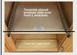
In the target cabinet opening lay the left and right cabinet rails into place parallel with each other, overlay the template between the rails aligning the front Lbrackets with the template's corner access holes.
