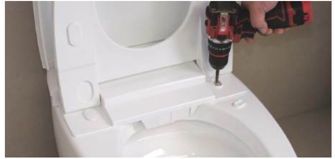
17. Reinstall and fix the positioning screws and the decorative cover.
