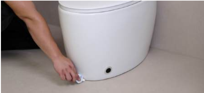
18. Apply some glass glue to fix the toilet and insulate the outside dirt from entering. ( The glass adhesive in the picture needs to be purchased by oneself. )
