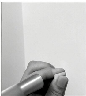
4. Install expansion nails in the holes
