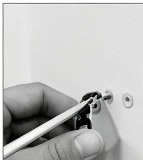
5. Install the clip on the expansion nails
