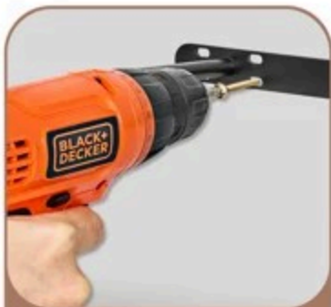
Attach Bracket to Wall
