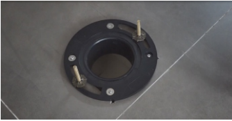
6. Install two long screws as below picture
