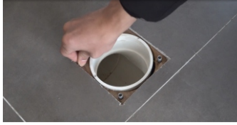
4. Put the screws into the holes
