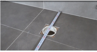
1. The confirmation of the installation environment, The measurement distance is 300mm or greater
