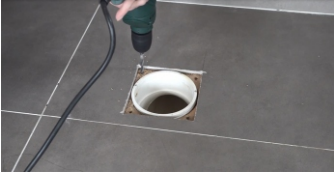
3. Take off the flange ring and drill four holes for screws
