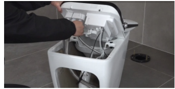
8. Take off the whole toilet seat and unscrew the flexible tube and black wire
