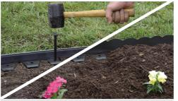
2 Hammer the included anchoring spikes through the tabs to hold the edging in place. The maximum spacing of the spikes is every 4'. If you desire additional anchoring, spike packs are available separately.
