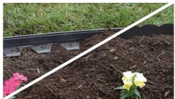
3 Backfill to the top of the edging with mulch or other groundcover.
