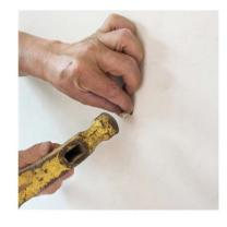
Step eight: Knock expansion pipe with hammer into the hole on the wall
