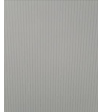
photo of the 4mm roof panel
