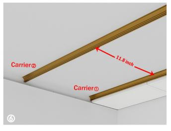
Then, install the second row of carrier② with screw 11.8 inch away from the carrier① (Center to Center).
