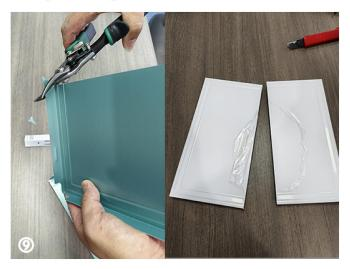
When the ceiling is installed to the edge  $\,(\,\mbox{end}\,)\,$  , the ceiling can be freely cut to fixed and complete the final installation.
