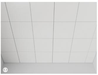
Repeat steps 6 and 7 until the second row of ceiling is installed. Repeat this way, install the carriers and ceilings of each row.
