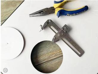
Note: the ceiling panel can be cut and opened according to the size of the lamp to install the lamp.
