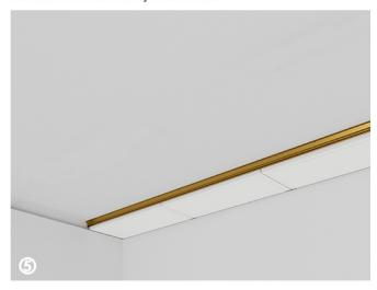
Continue to install the first row of carriers, and repeat steps 3 and 4 until the entire row of ceiling is installed.
