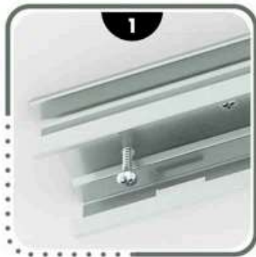
Install the top track
