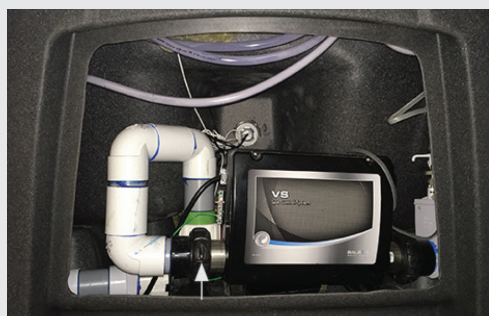
FIGURE 1.5A -- HEATER UNION; LOOSEN UP TO BLEED AIR
