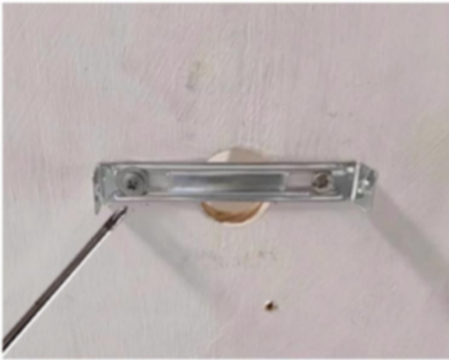
3. Secure the mounting plate Secure the mounting plate to the ceiling with self-tapping screws.
