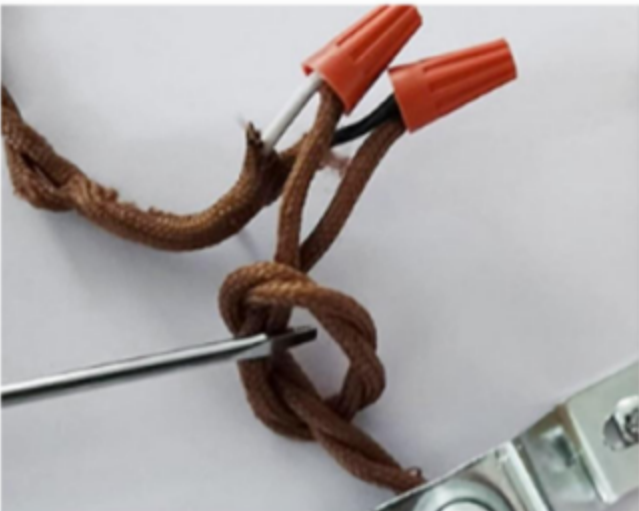
5. Connect wires 1. Adjust the length of the light cord. 2. Tie a safety knot on the hanging board. 3. Connect the wires with wire caps or electrical tape.
