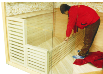
FIG-13 Assembling sitting board's support
