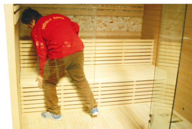
FIG-14 Assembling sitting board's support
