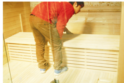
FIG-12 Assembling sitting board's support
