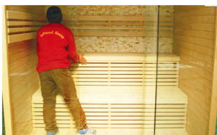
FIG-15 Assembling sitting board
