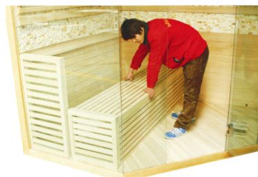
FIG-14 Assembling sitting board
