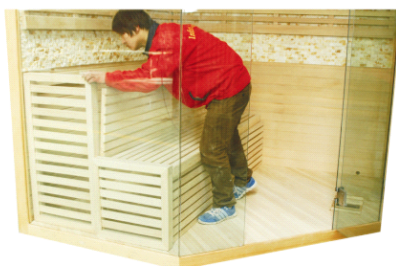
FIG-15 Assembling sitting board's support
