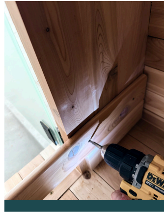
18. Open the door and remove the interior supports.
