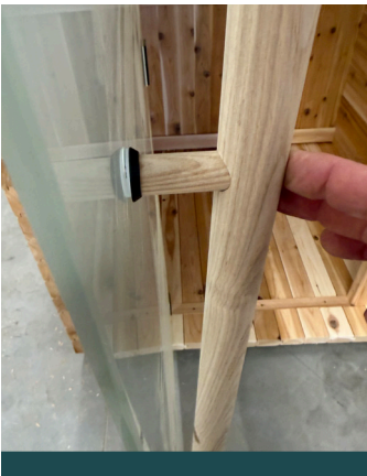
20. Insert the screw from the handle through a hole in the glass to attach the opposing handle. Be sure to place the metal handle on the outside of the changing room and the wood handle in.
