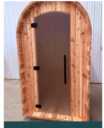
23. Completed changing room with door hardware installed.
