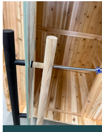
22. Tighten the screw to pull the handles together against the glass. Attach all handle fittings before tightening.
