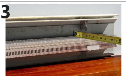
Measure from the back plate to the front of the heating element.
