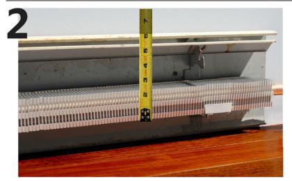
Measure from the bottom of the heating element to the top of the existing back plate.
