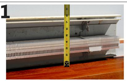
Measure from the finished floor to the top of the existing back plate.
