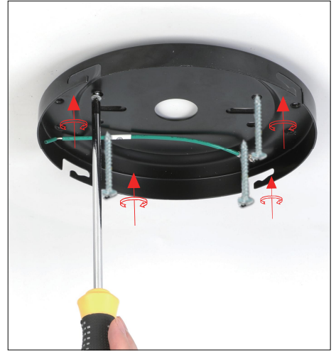
For the wood ceiling: Start by marking the location for the ceiling fan. Then, use the 4 wood screws provided to securely attach the mounting bracket to the building structure.
