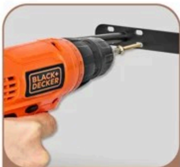
Attach Bracket to Wall
