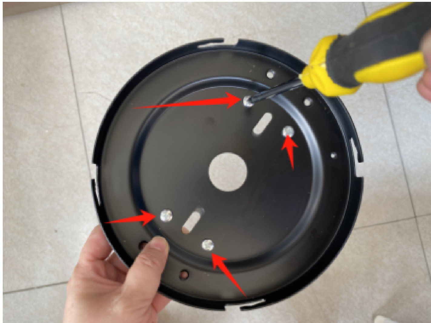
Ceiling Bracket mount to wood ceiling
