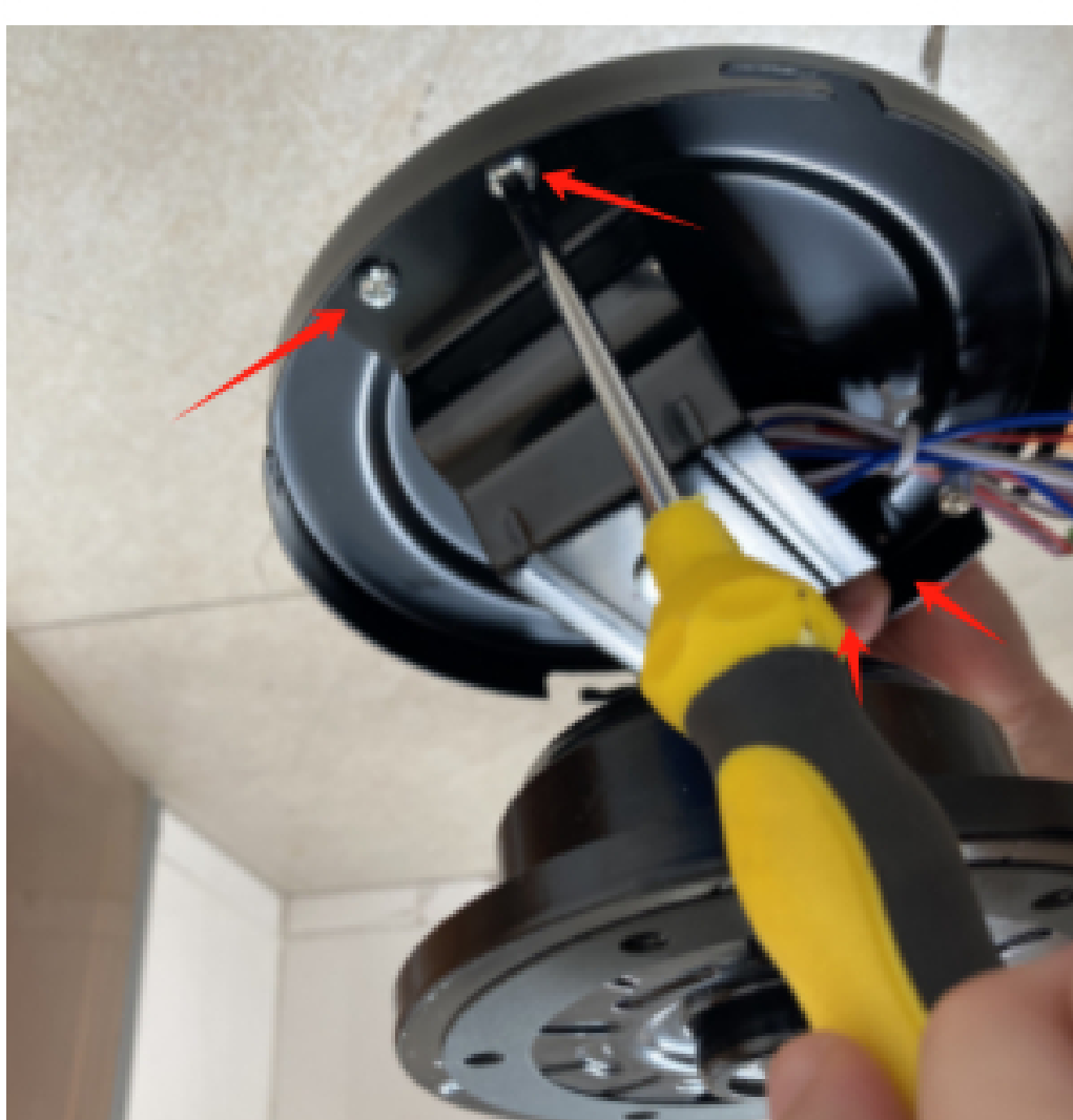
Hang the motor to the ceiling bracket
