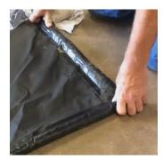
STEP 2 Position the AFG mat on the floor where you want it; starting with the edge nearest to the garage door.
