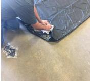
STEP 3 Mark the floor with chalk or tape (not included) around the corner edges of the AFG.
